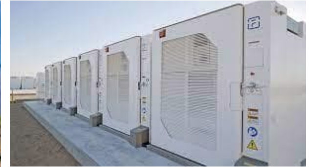
2.75MW/5.5MWh, BESS Installation
